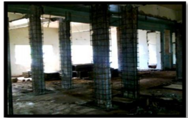
Fig1: Jacketing of column
