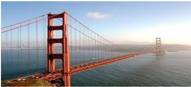
Fig No.1 Bridge with Suspension
